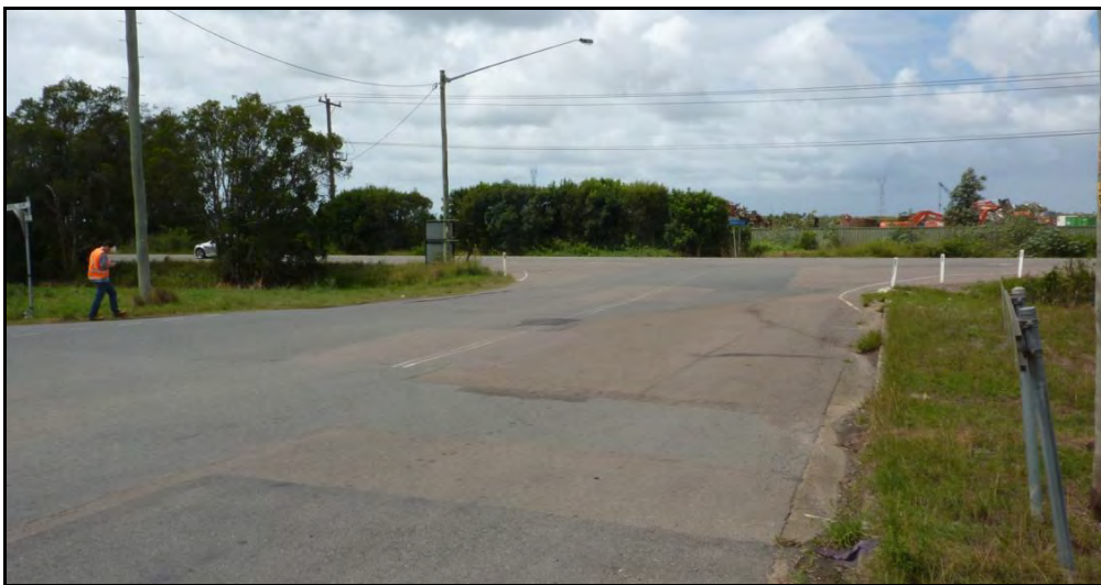
Figure 14.4 McIntyre Road (looking towards Tomago Road)
