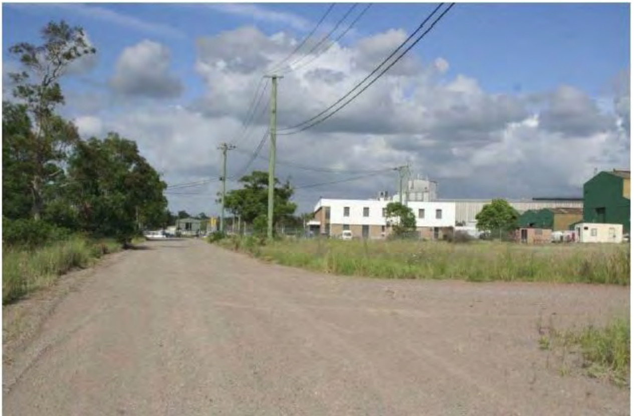
Photo 4.2 Existing gravel roads providing access to the site
