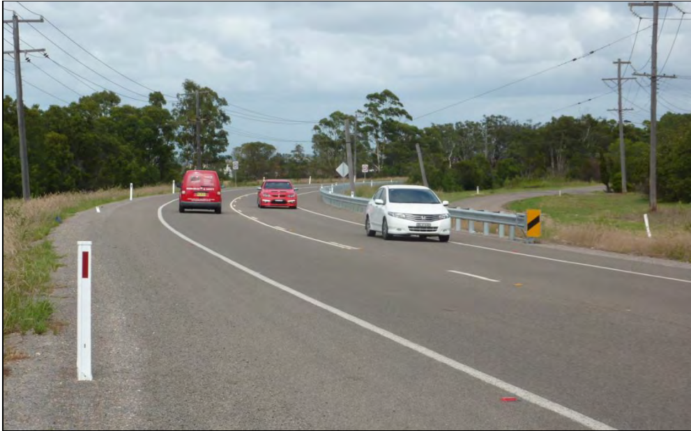
Figure 14.3 Tomago Road (looking west towards approach to McIntyre Road)
