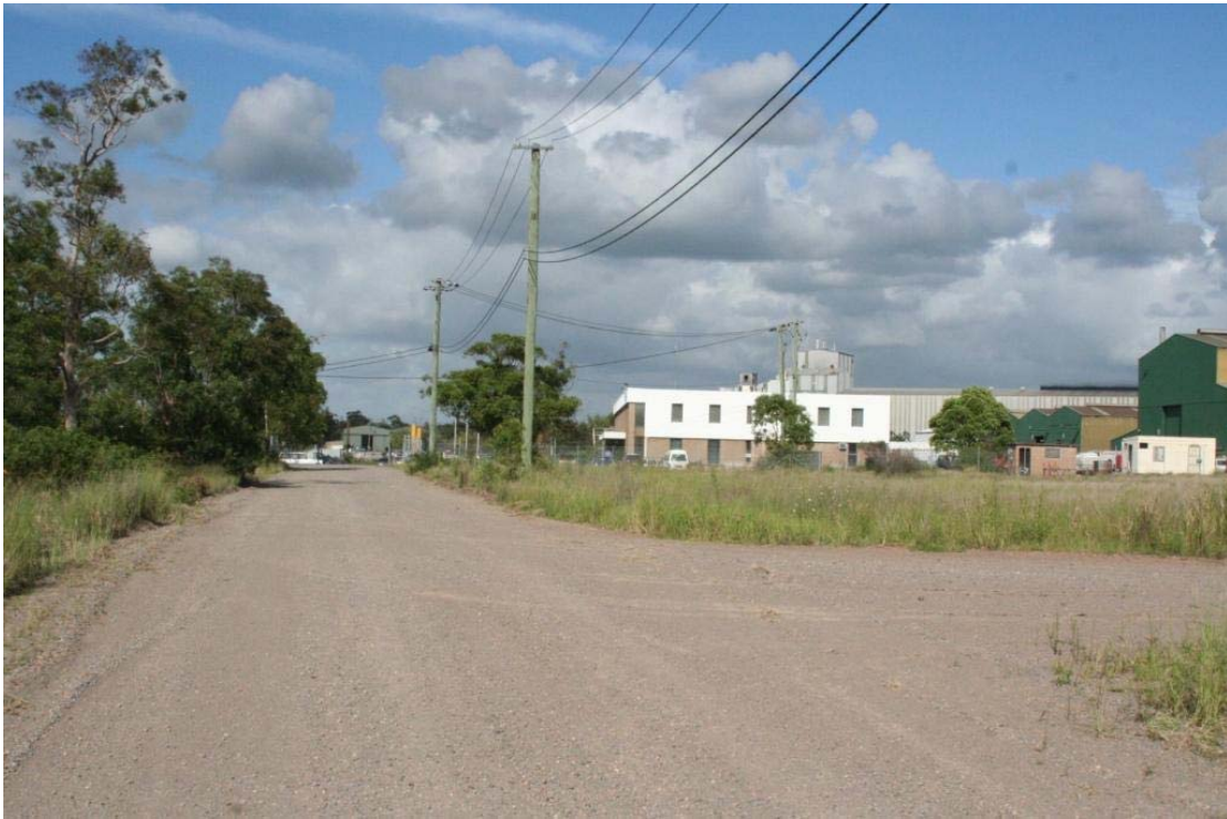
Photo 3 Existing gravel roads to be rebuilt and sealed
