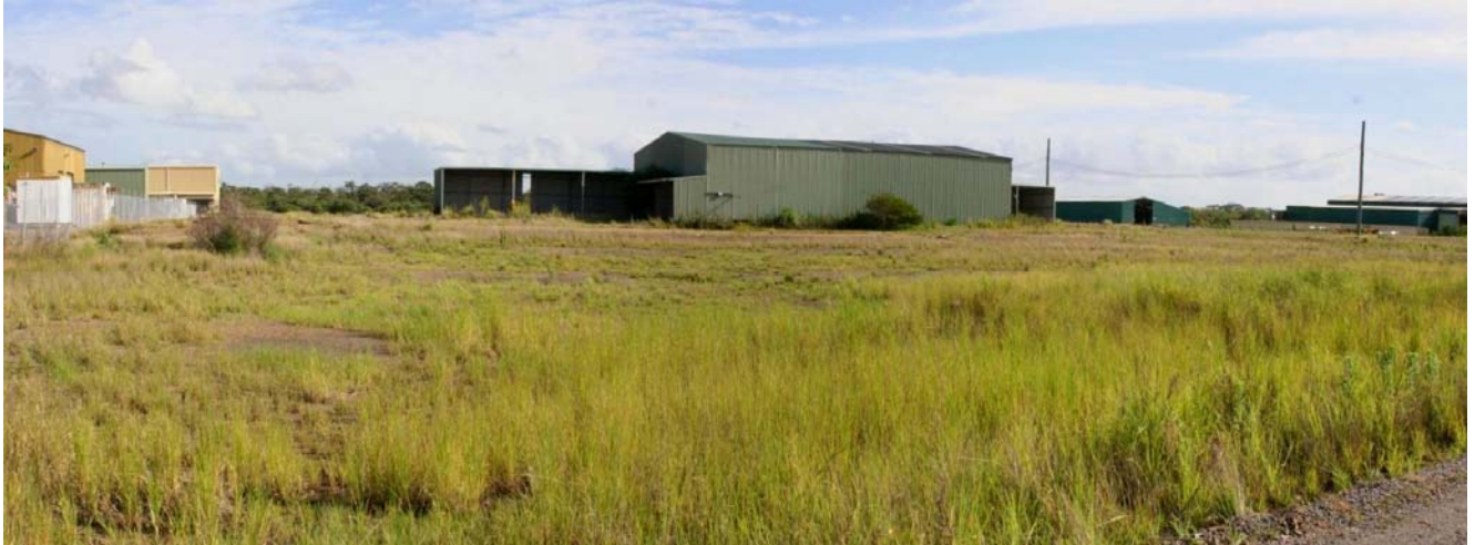
Photo 1 Proposed Site looking north showing the existing building
