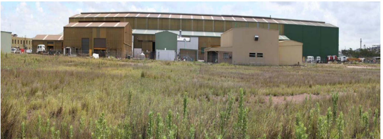
Photo 2 Existing industrial development adjacent to the site to the west
