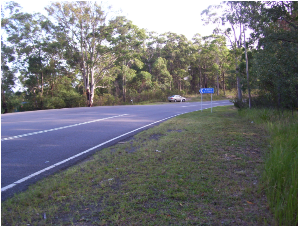
Figure 6-1 Eastern verge showing substandard shoulder and tree in 'clear zone'
