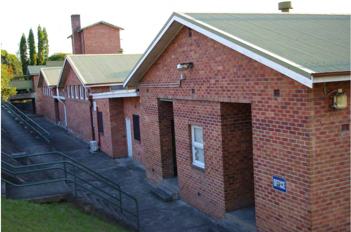
Plate 6-2 Awaba administration buildings, built c1950
