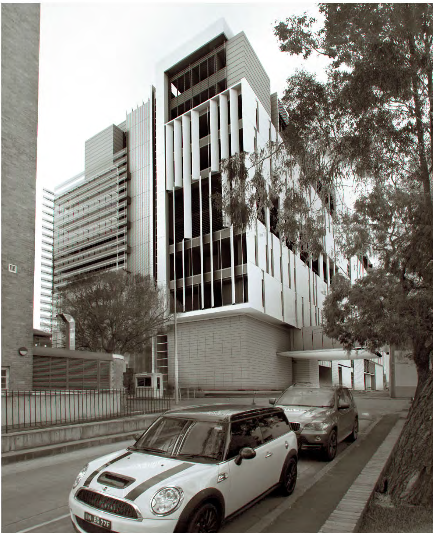
NORTH WEST VIEW
