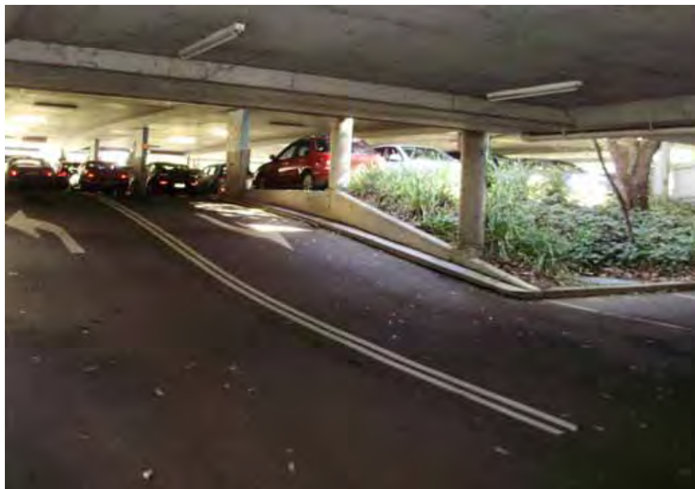
Photo 15: Car park ramp leading down from W1 to W2
