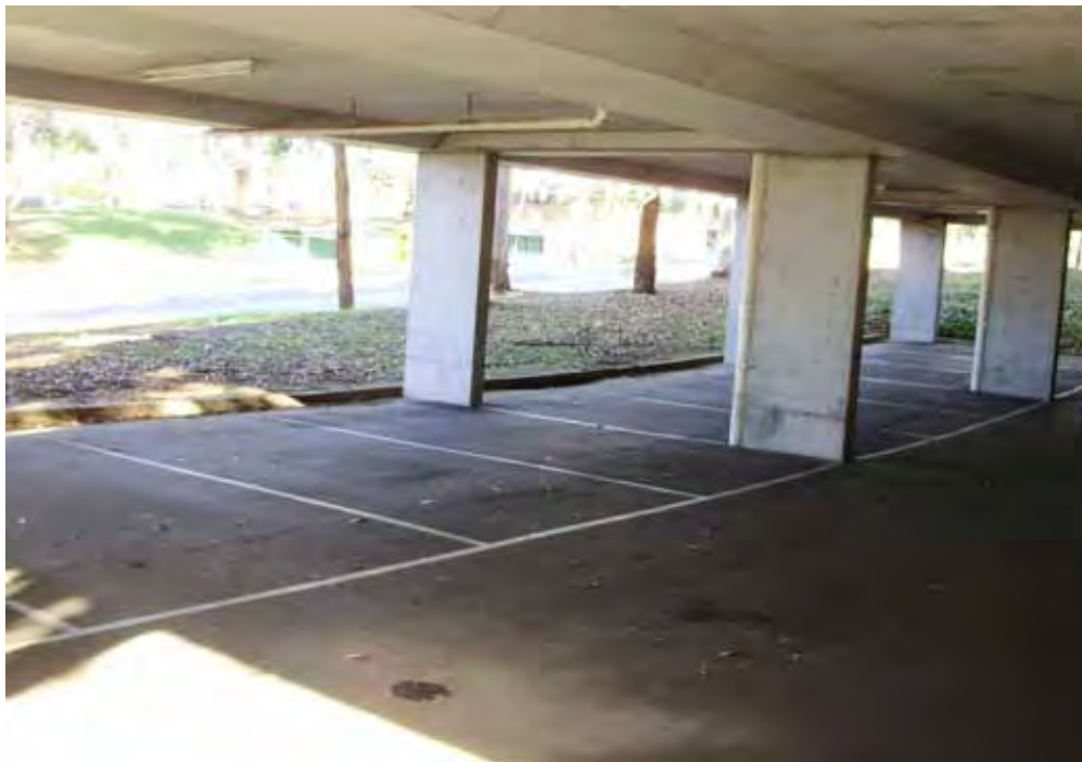
Photo 14: BH16 within car park W2 facing south towards University Avenue
