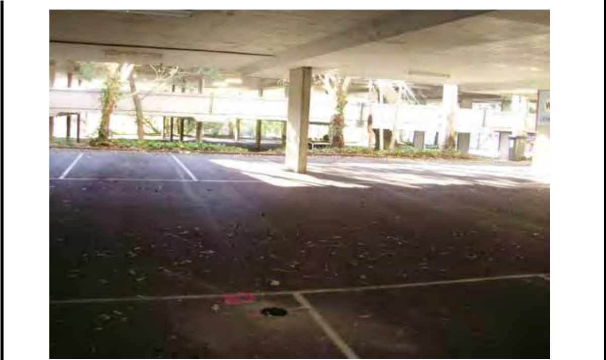
Photo 13: Location of BH15 within car park W2 facing east towards C1 car park
