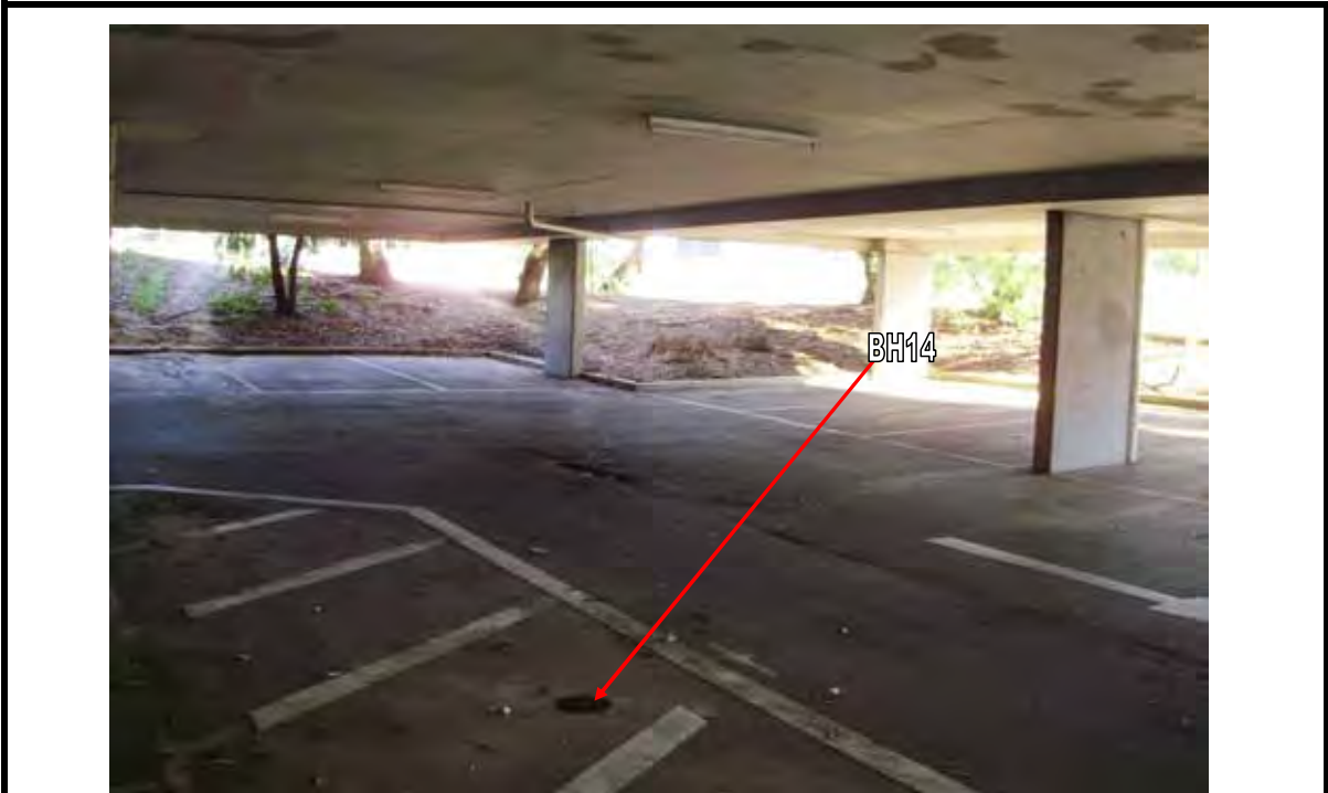
Photo 12: BH14 located within car park W2
