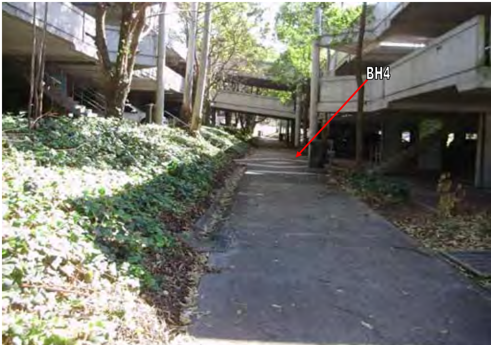
Photo 5: Walkway along eastern boundary of subject site (W2 car park) and C1 car park
