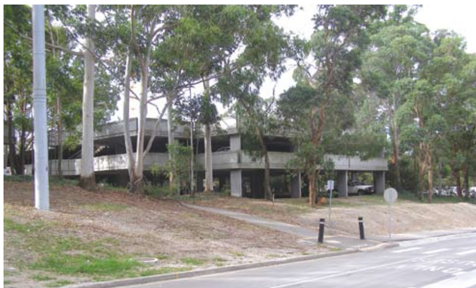
Figure 5 – View of carpark C1 from University Avenue
