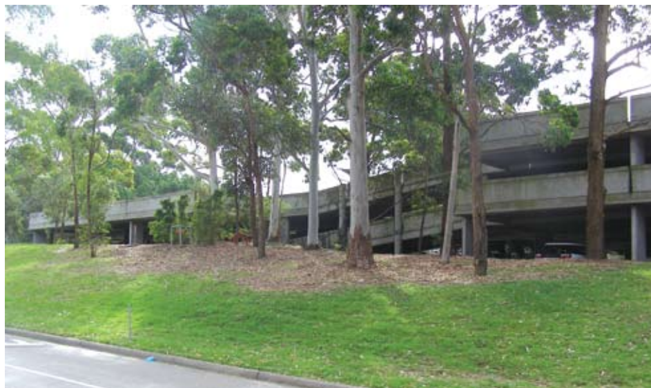
Figure 6 – View of carparks W1 and W2 looking north-west
