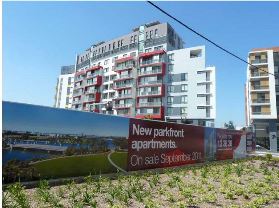
Figure 4 – Existing hoarding around Stage 2
