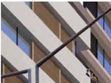
Northern apartment spandrels Painted precast concrete
