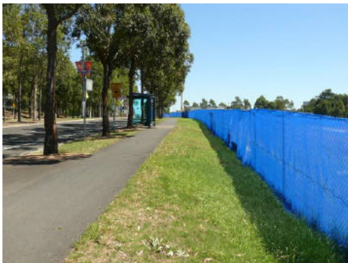
Figure 7 Australia Avenue site frontage Australia Avenue is the main frontage to the site
