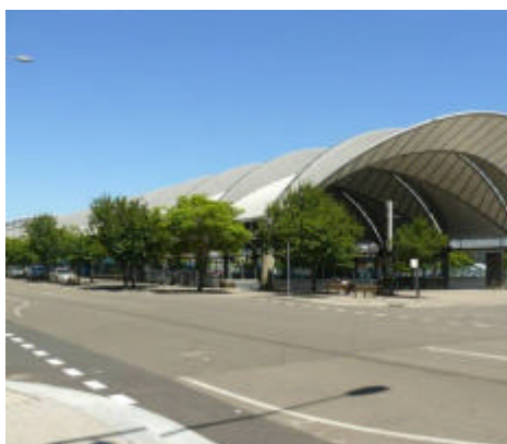
Figure 11 Sydney Olympic Parktrain station Located on Dawn Fraser Avenue approximately 250 metres from the site
