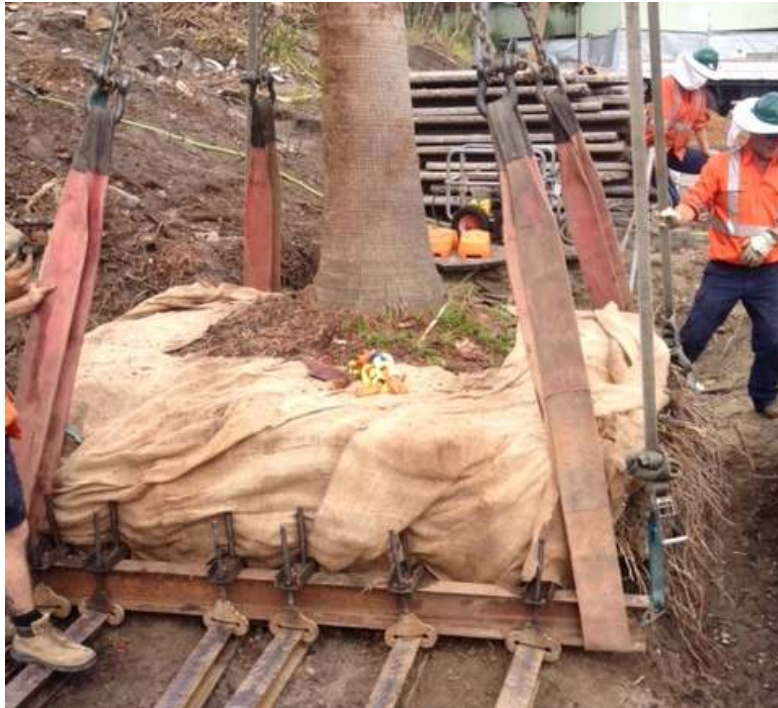
Figure 1: Prepared root plate being lifted from original location
