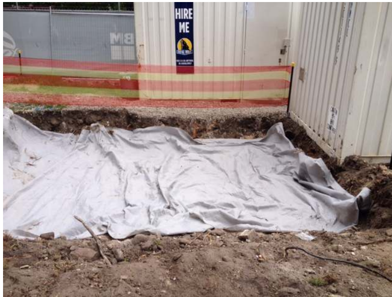
Figure 2: Temporary Location prior to installation of tree (approx 10m 2 )
