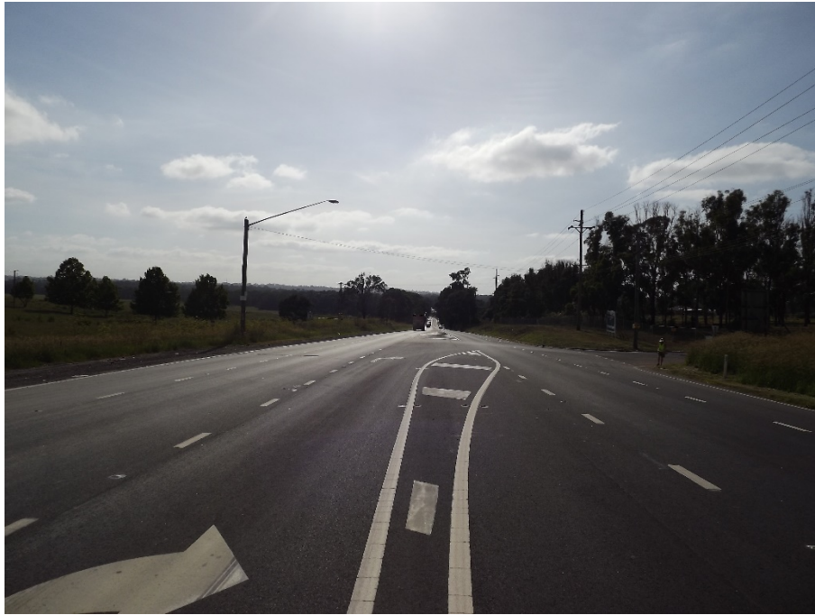
2. Elizabeth Drive eastbound approach
