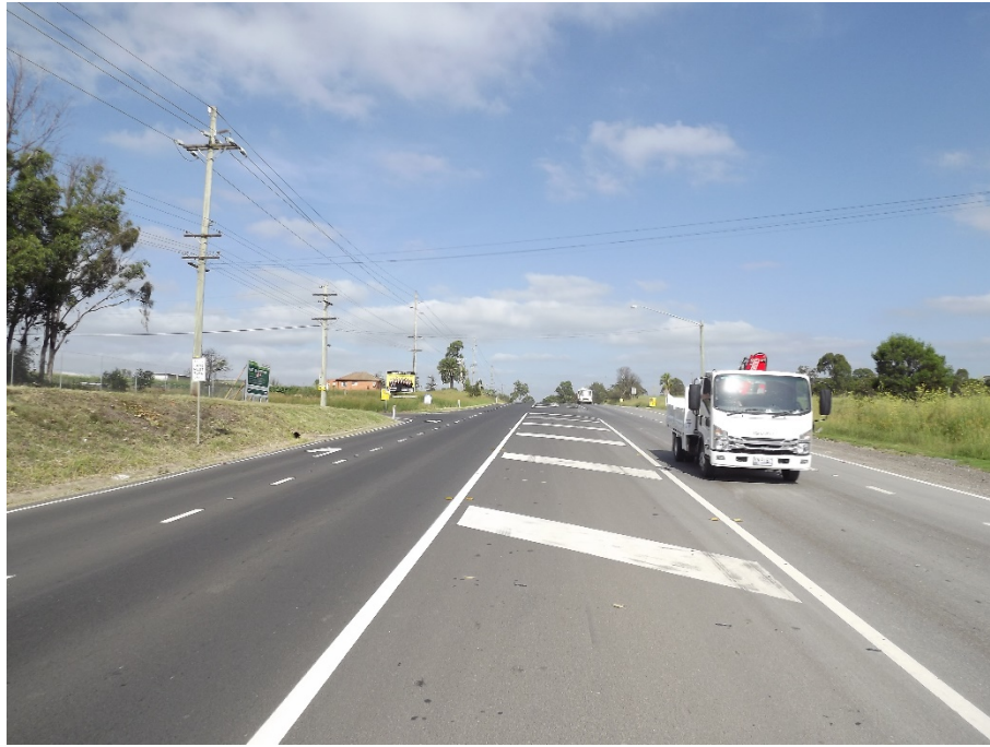
3. Elizabeth Drive westbound approach
