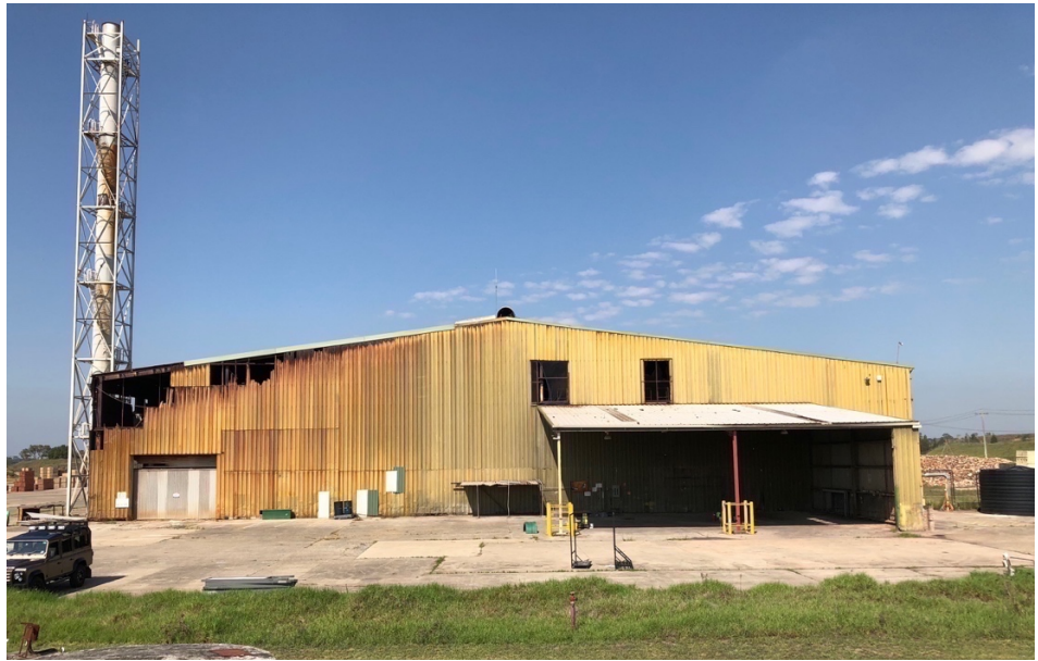
FIGURE 3.5: CENTRAL HARDSTAND YARD AND BRICK MAKING FACILITY 10
