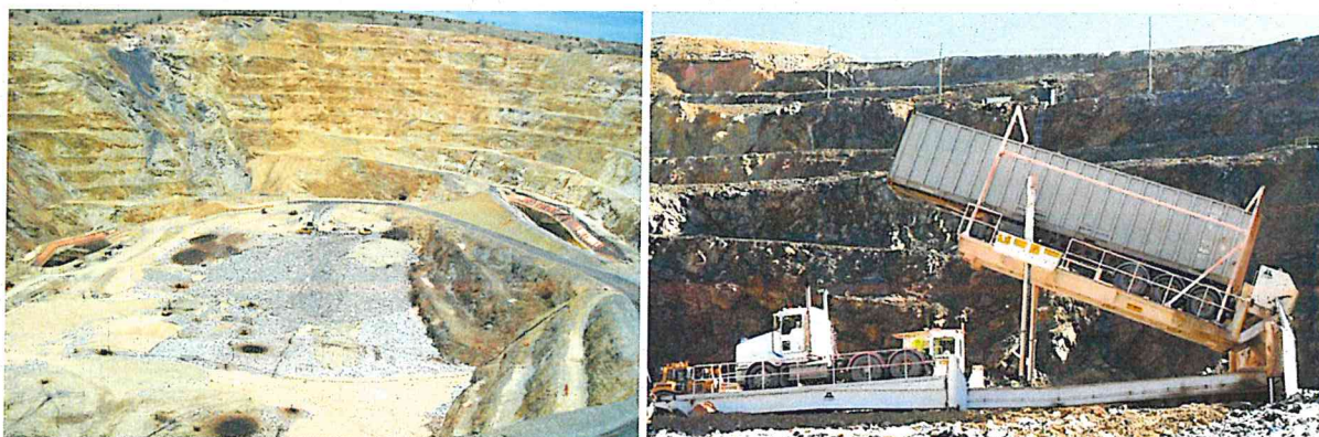
Figure 5: Woodlawn Bioreactor void and waste container tipping area
