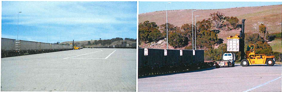
Figure 3: Crisps Creek IMF hardstand and container unloading area
