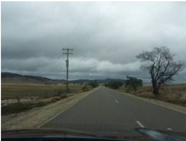
Plate 2-1 Collector Road, Towards East, East of Woodlawn Bioreactor Access
