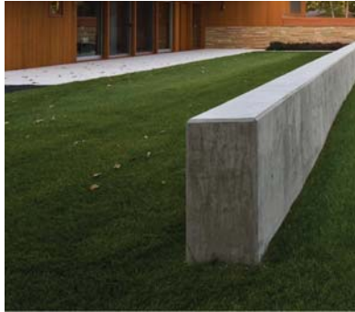
Concrete Blade walls
