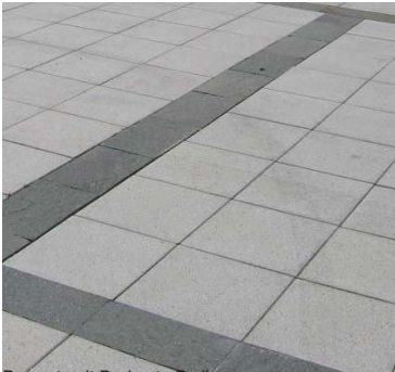
Precast unit Paving to Podium.
