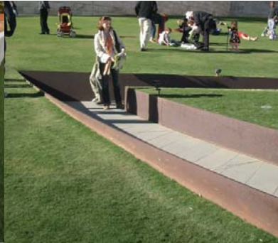
Coreten Steel walls to turf edges
