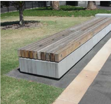
Concrete block bench seating
