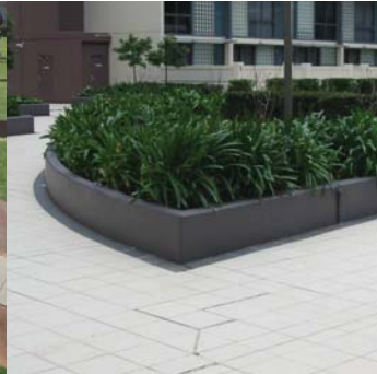
Rendered blockwork planter to podium planters
