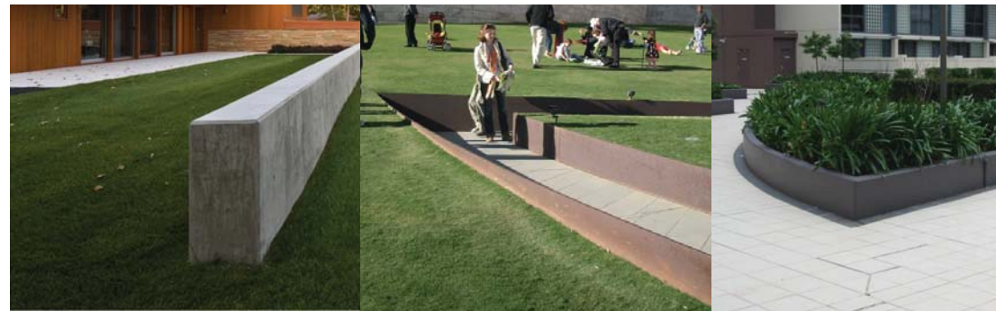
Concrete Blade walls Coreten Steel walls to turf edges Rendered blockwork planter to podium planters
