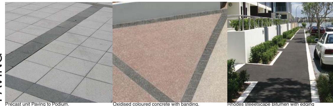
Precast unit Paving to Podium. Oxidised coloured concrete with banding. Rhodes streetscape Bitumen with edging
