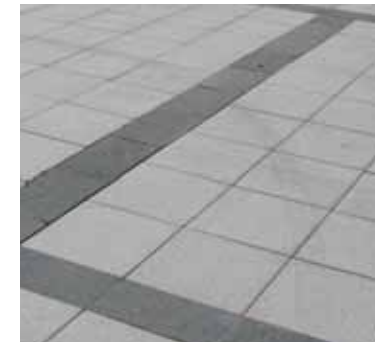
Precast unit Paving to Podium.
