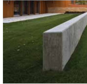
Concrete Blade walls
