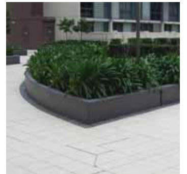
Rendered blockwork planter to podium planters
