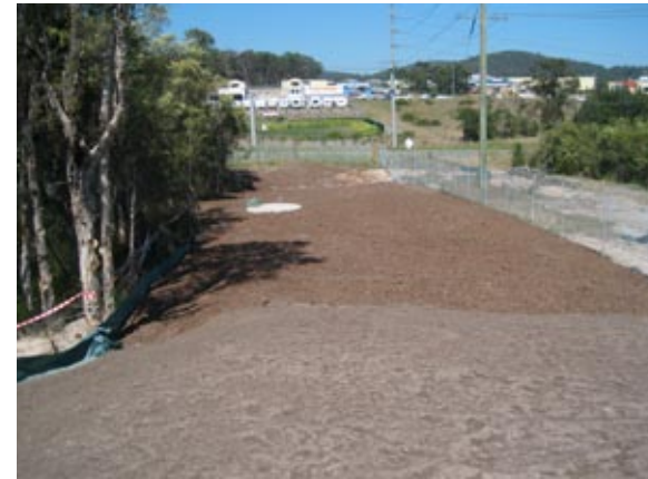
PHOTOGRAPH 3: Soil Spreading.
