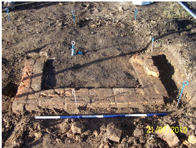
Figure 2.7 Detail of the fireplace footing and part first fireplace course, MH11-E, from north. Paul Rheinberger Scale: 200mm
