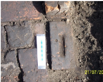
Figure 2.15 Detail of two identifiable brick types in the apron, MH5-E: At left, a brick and batt with heart shaped frogs of 'The Pack' type; at right, the long semi-round ended rectangular frog of the early Maitland style. Paul Rheinberger Scale: 10mm
