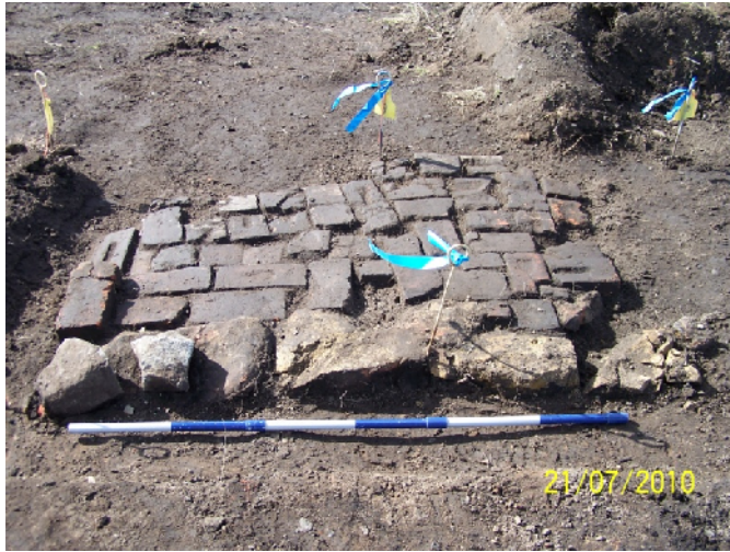
Figure 2.13 Detail of the door sill and brick and brickbat apron, MH5-E, from west. Paul Rheinberger Scale: 200mm
