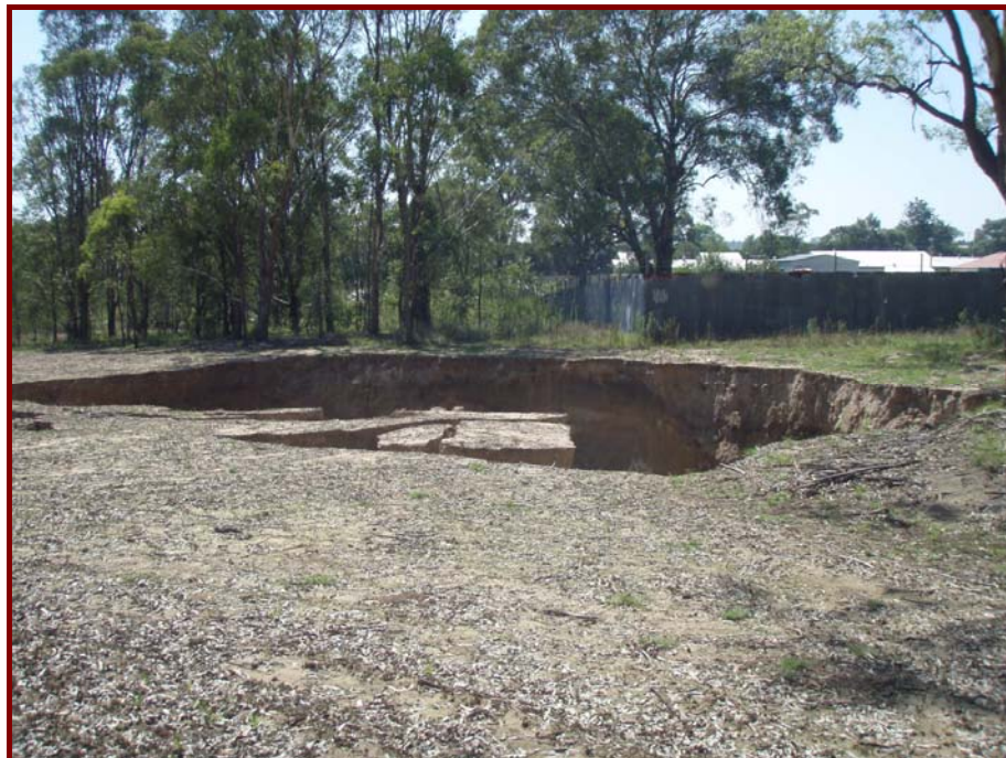
Plate 5 - Large pothole towards southern end of the site, February 2009 Photo provided by the MSB
