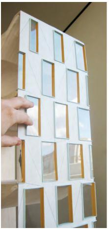
Typically the windows are positioned in a 350mm deep frame. The depth of this frame takes up the dimension of the varying vertical and horizontal facade undulation.
