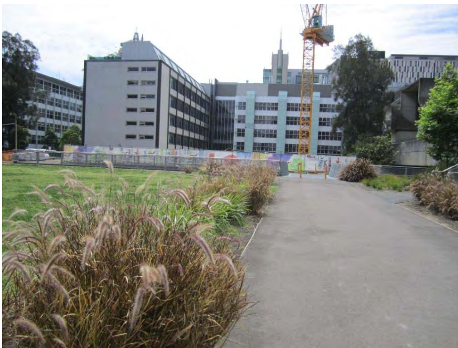
Jones Street north of Building 2 looking east
