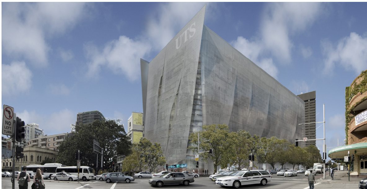
Figure 9 - Building identification signage on Broadway and Wattle Street (Source: DCM)
