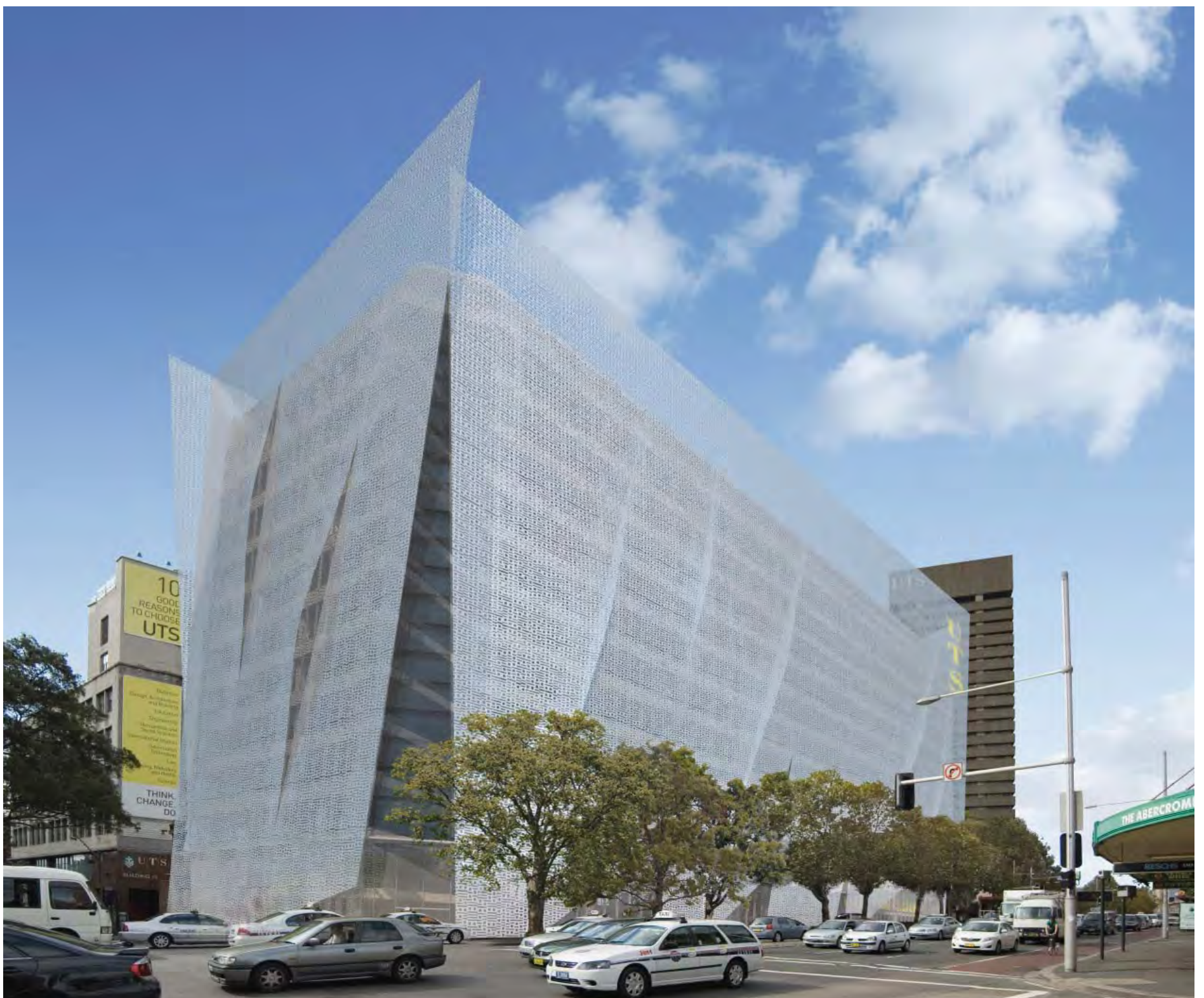
Visual Impact view corner Broadway and Wattle Street: Plant and roof mounted equipment is concealed.
