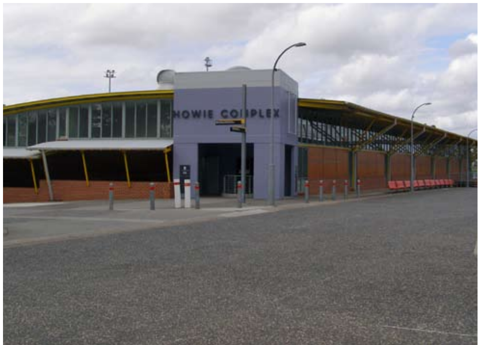
Figure 12 – Howie Complex as viewed from Riverina Avenue
