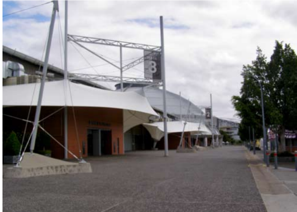
Figure 4 – Northern elevation of the Exhibition Hall looking west
