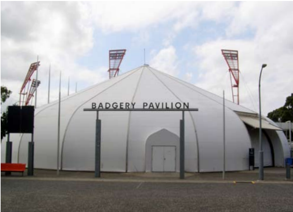
Figure 10 – Badgery Pavillion as viewed from Riverina Avenue
