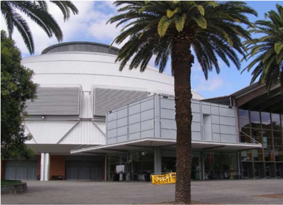
Figure 6 – Western elevation of the Dome Building
