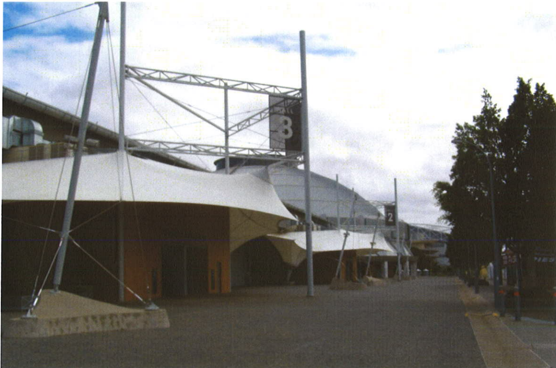
Figure 2 – Northern elevation of the Exhibition Hall looking west
