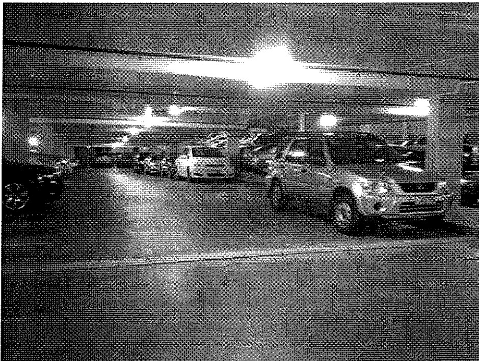
Photograph ii. Promontory Car park showing parking onto ramps due to overreaching capacity, Level 2. December 7, 2010.
