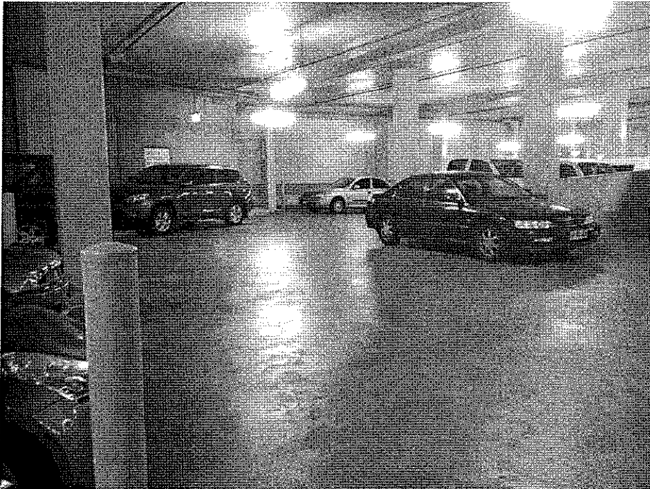
Photograph iii. Promontory Car park showing parking on corner of thoroughfare, Level 3-4. December 14, 2010.
