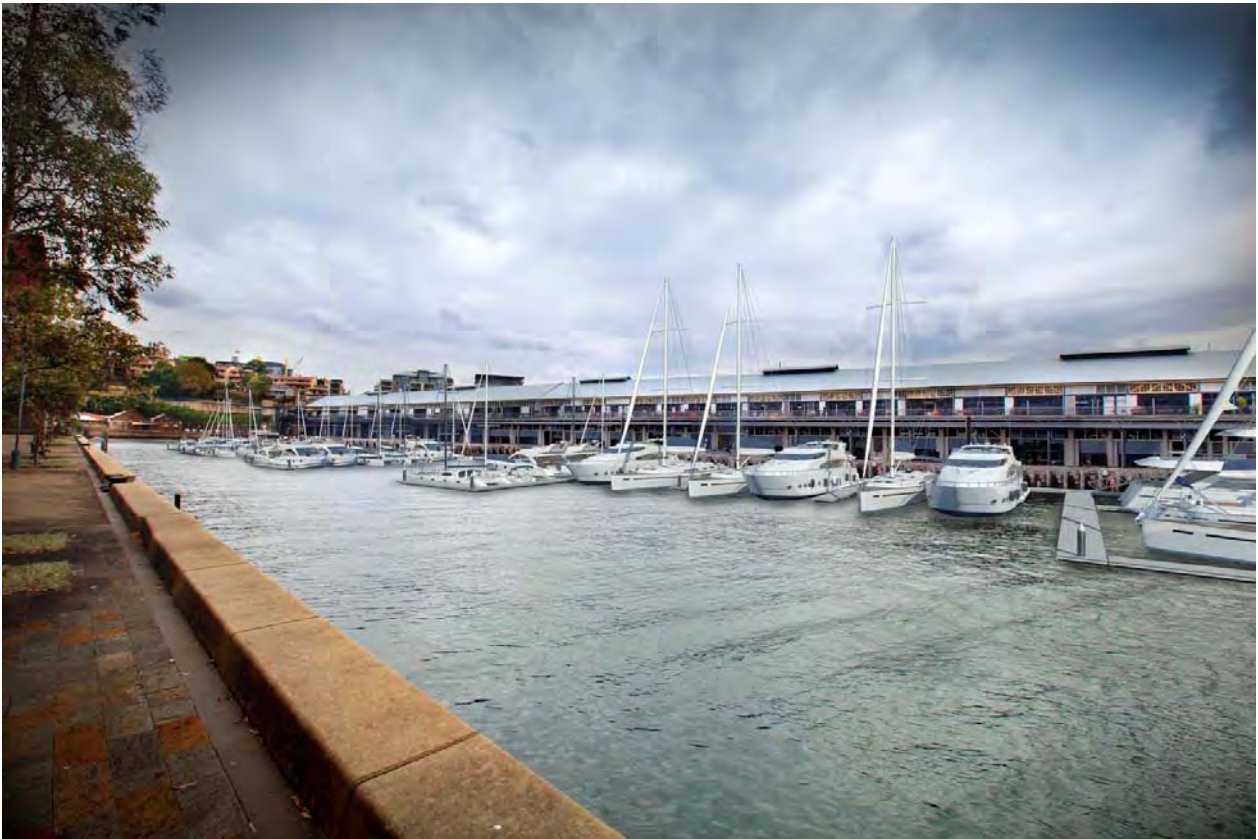
Figure 12 - View 10 – Looking south west from public foreshore promenade across the eastern side of Jones Bay towards Pirrama Road.
