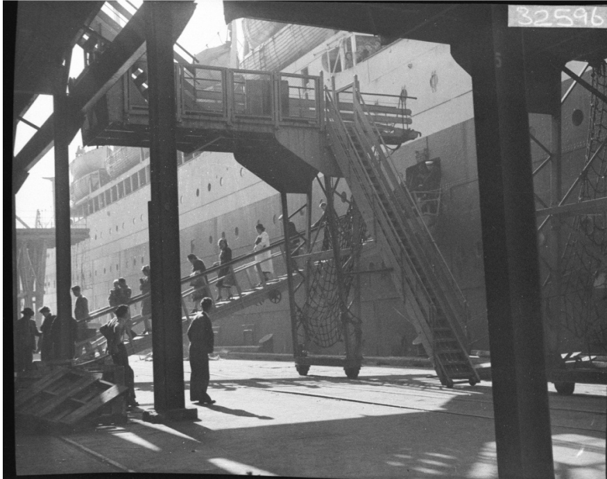
Ships berthed at Jones Bay Wharf date unknown, probably 1930s.
