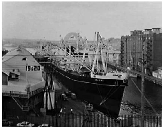
Figure 2 – Large vessel alongside the eastern side of Jones Bay Wharf
