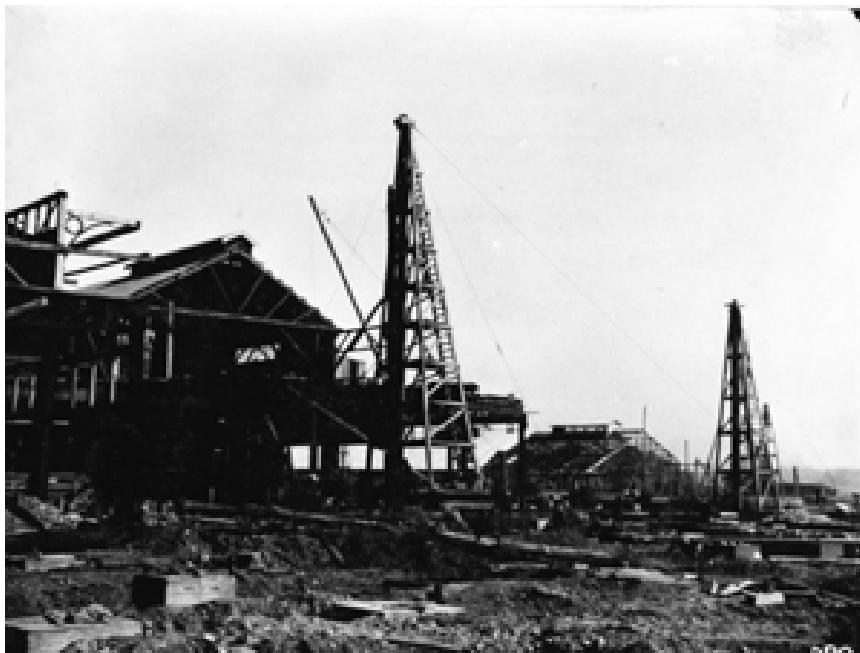
Fig 4.4 Construction of Jones Bay Wharf showing pile drivers 1917. Source: ML GPO 1-21194.
