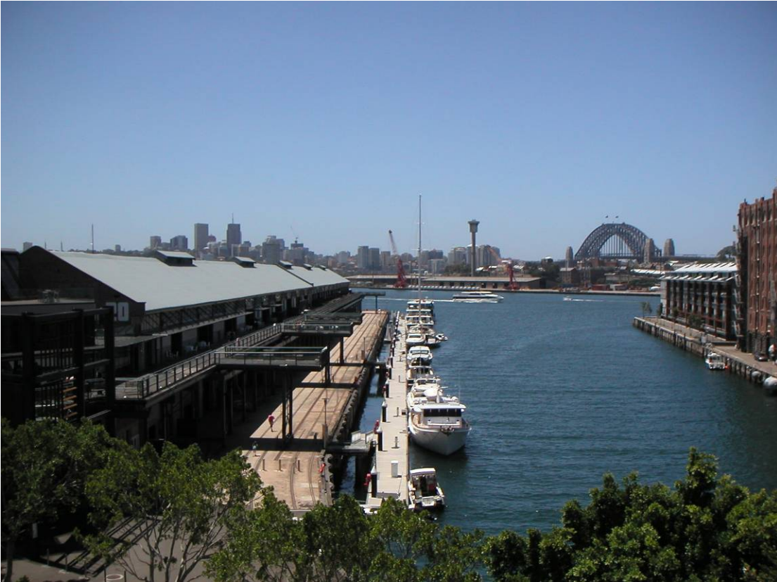
Figure 4 – Jones Bay Wharf Marina existing pontoons eastern side
