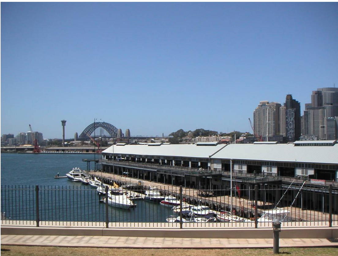
Figure 6 – Jones Bay Wharf looking north-east towards Sydney CBD
