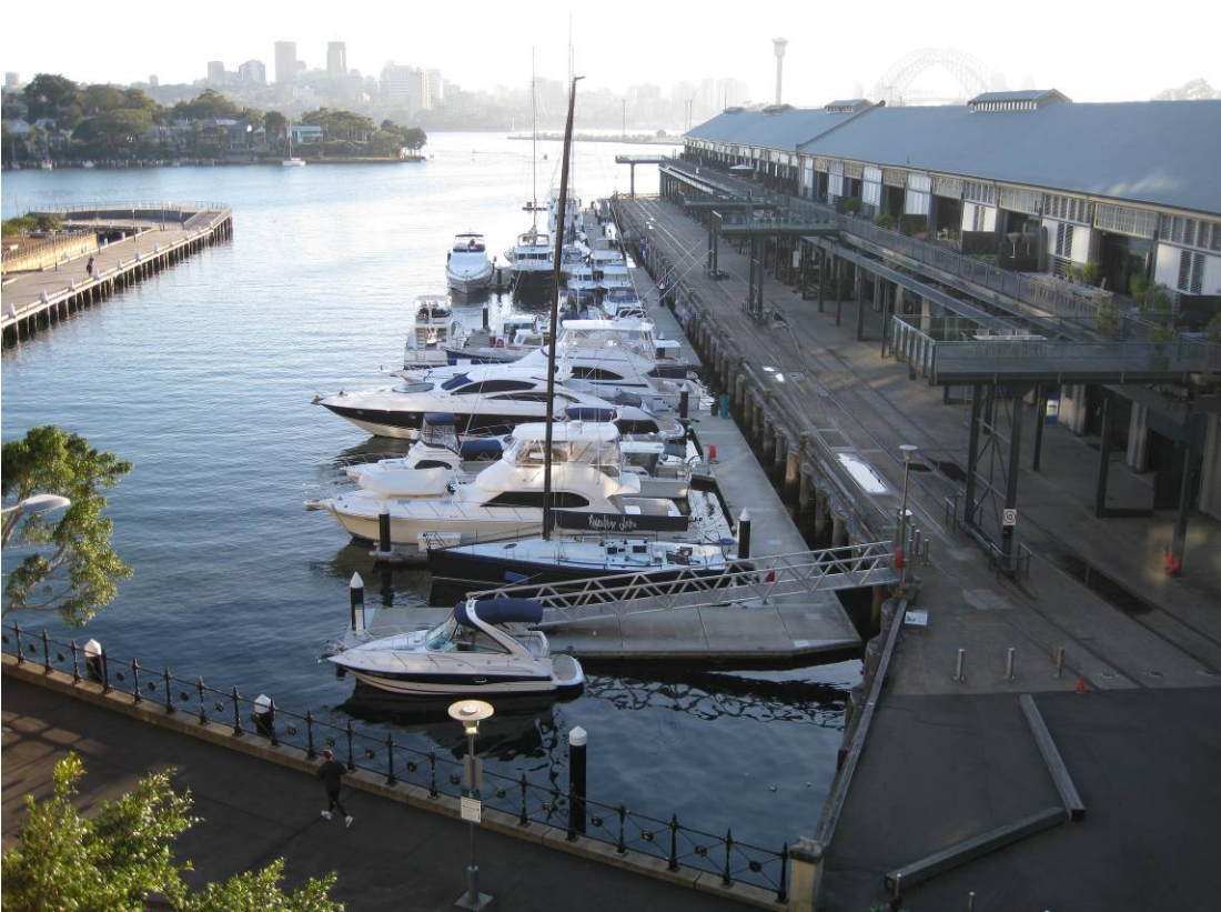
Figure 5 – Jones Bay Wharf Marina existing pontoons western side (private marina in foreground)
