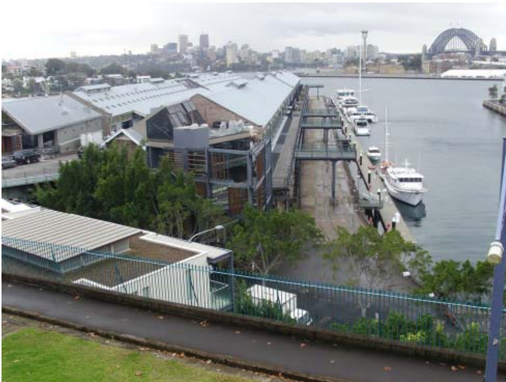
Figure 3. The existing marina on the eastern side of the wharf has a parallel floating pontoon only.
