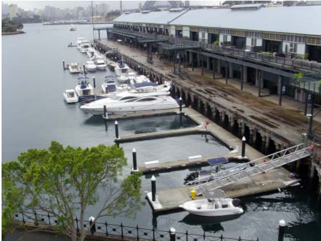
Figure 2. The existing marina on the western side of the wharf has both parallel and right-angled floating pontoons.
