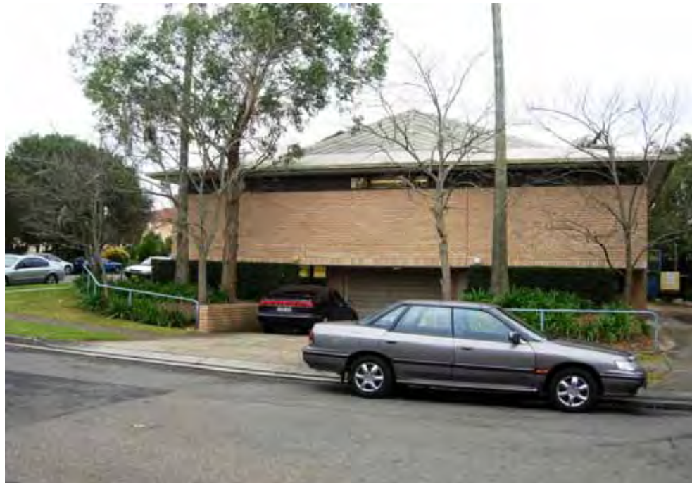
Photo 11: Rear of San Day Surgery from Balmoral Street facing east
