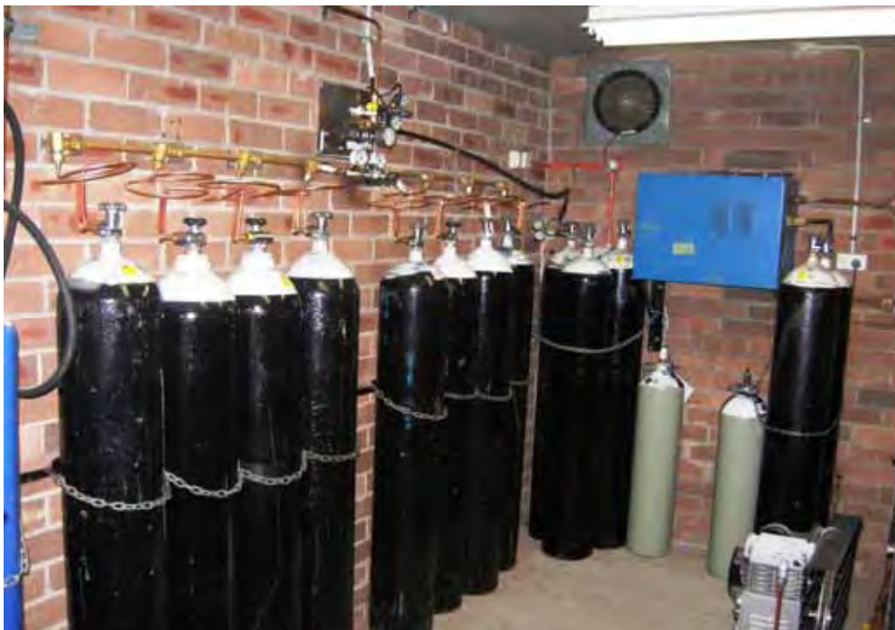
Photo 17: Non-flammable gas store room within basement of Surgery
