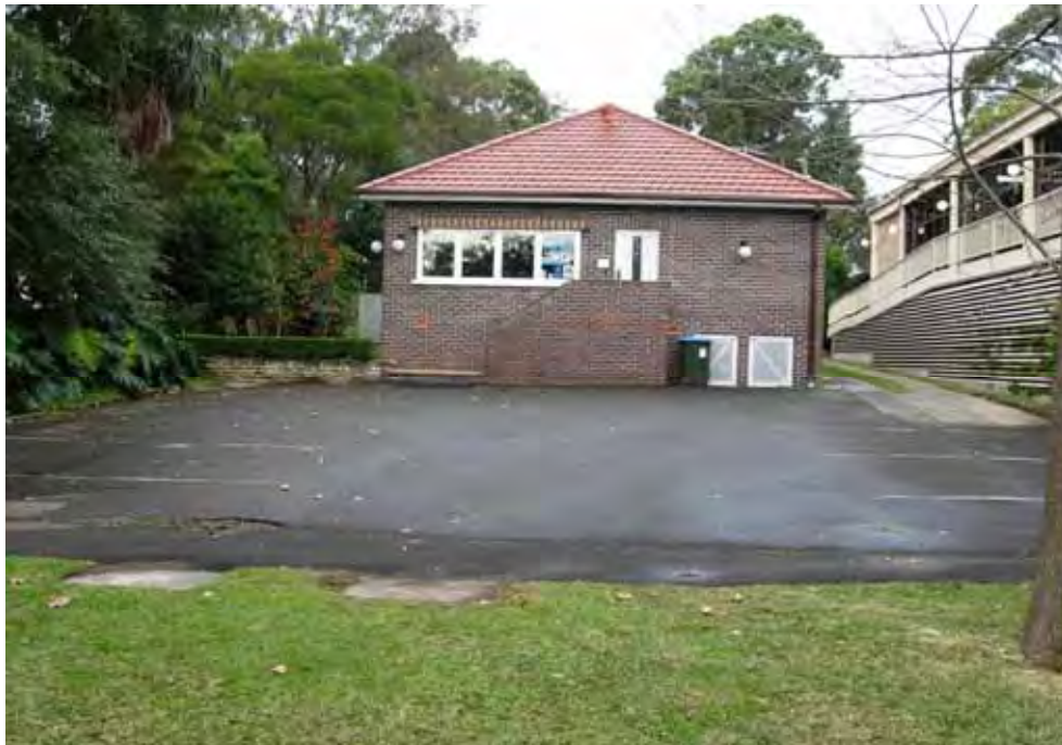
Photo 2: The rear of 55 Palmerston Rd facing east
