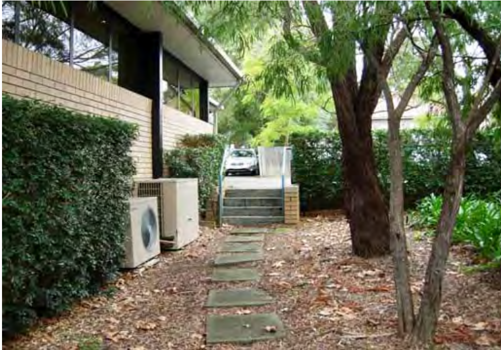
Photo 12: Southern side of San Day Surgery building facing car park to the east
