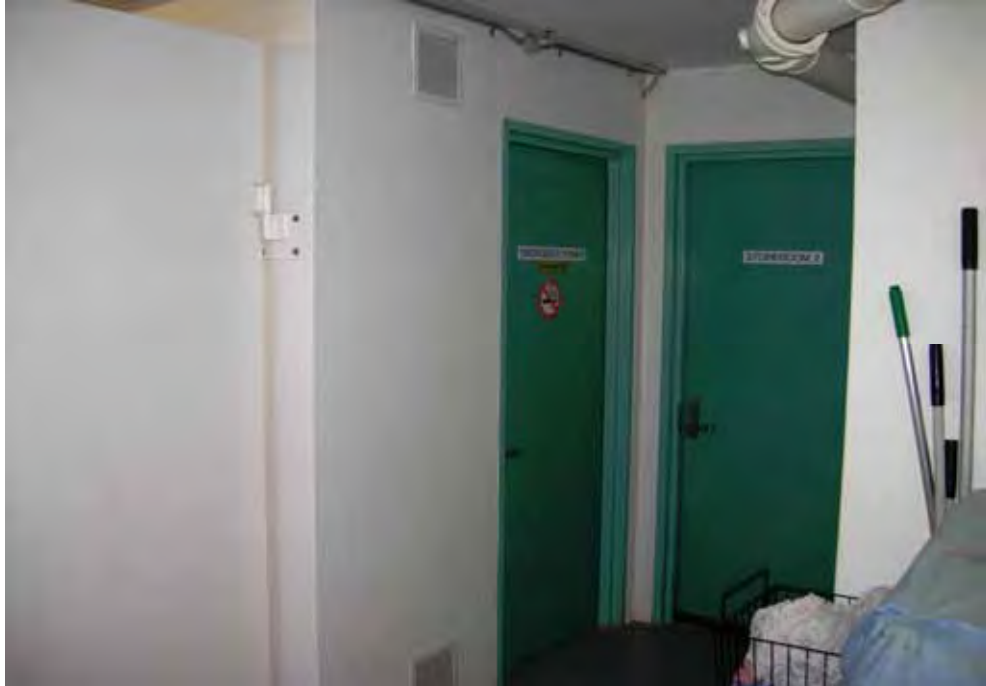
Photo 14: Surgery basement level comprising of waste collection, power room, store room and gas store
