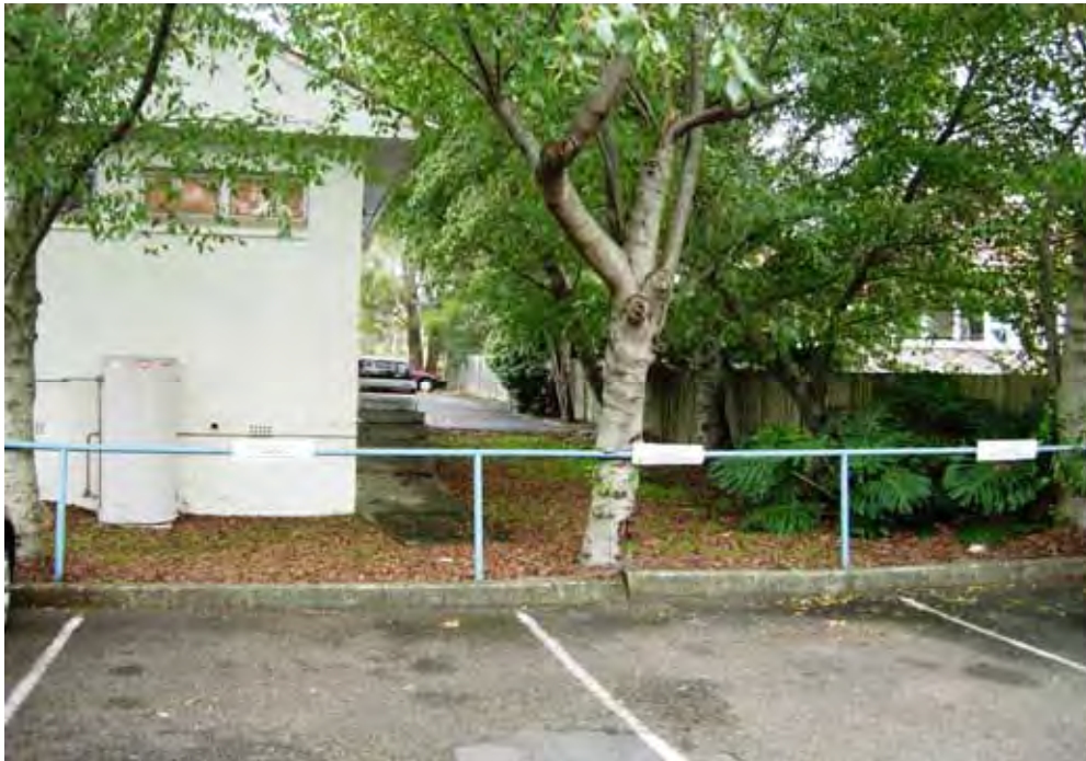
Photo 7: Rear of 57a Palmerston Rd from car park of the San Day Surgery
