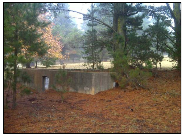
Figure 4.16 View of concrete cellar at HSPH5, looking south
