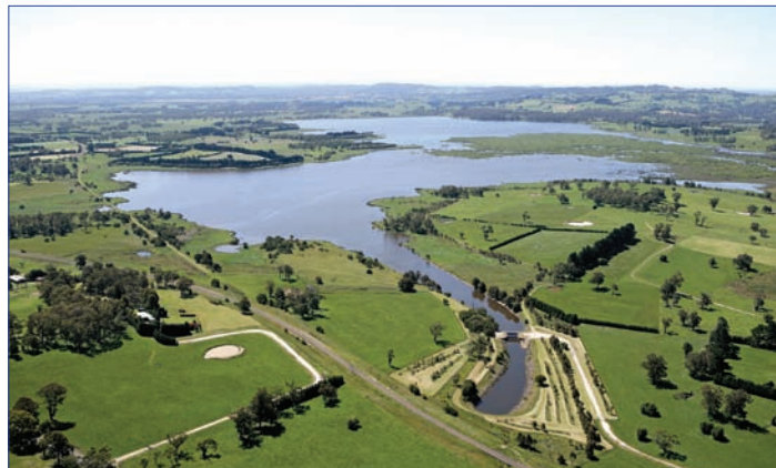
The Highlands Source Project, linked to Wingecarribee Reservoir (above) will provide a more reliable water source to the NSW City of Goulburn, which has a population of around 22,000 people.
