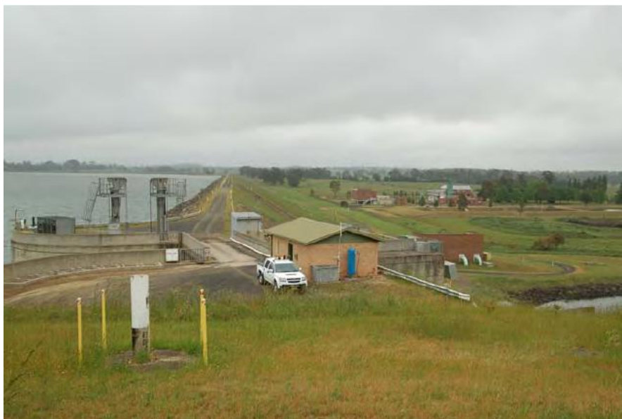
Figure 17.1 The existing pump station located at the Wingecarribee Reservoir.
