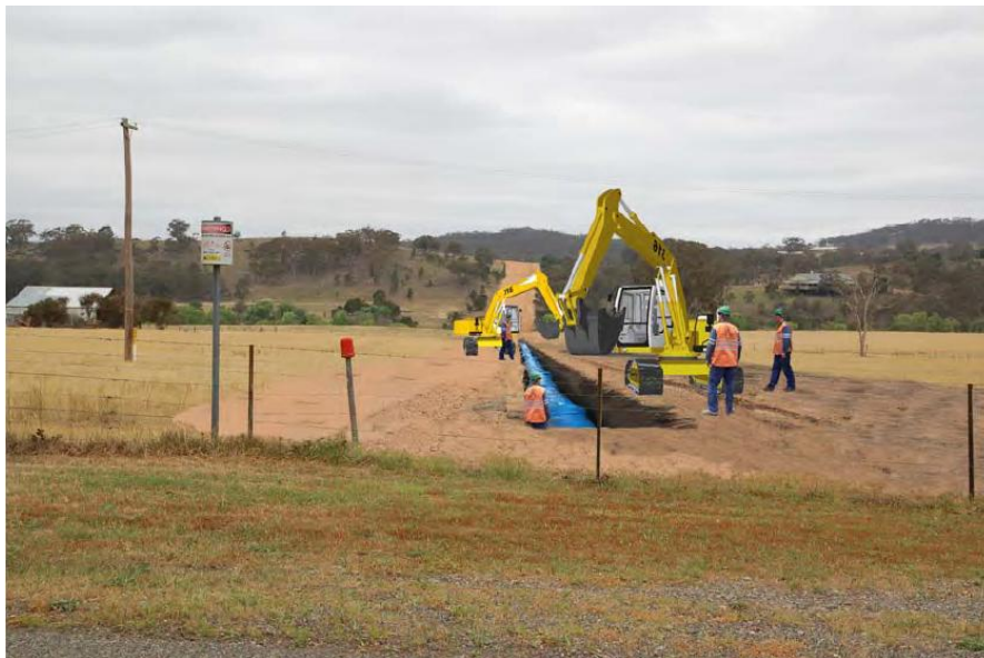
Figure 17.5 Indicative photomontage visualisation showing construction phase works from Towrang Road
