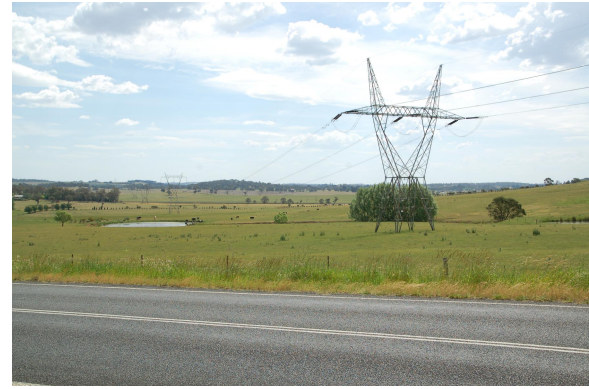
2. Werai-Moss Vale (View west from Mount Broughton Road. Proposed pipeline alignment follows powerline easement)
