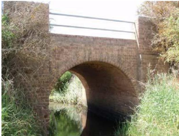
Figure 12.3 Brick bridge at HSPH2, looking southeast
