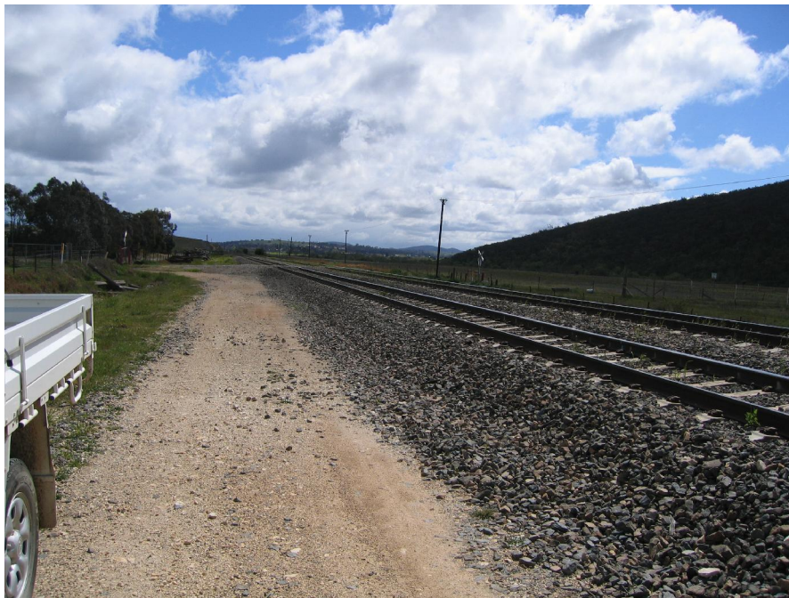
Figure 6.20 Main Southern Railway crossing point No. 3
