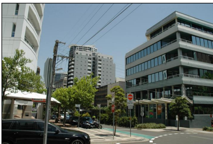
Photo 3: View of the site from Mitchell Street
