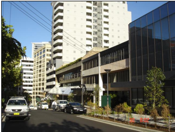
Photo 1: Atchison Street frontage looking west
