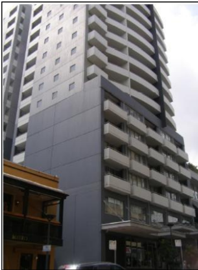
Photo 4: No. 2-4 Atchison St, Linea Building
