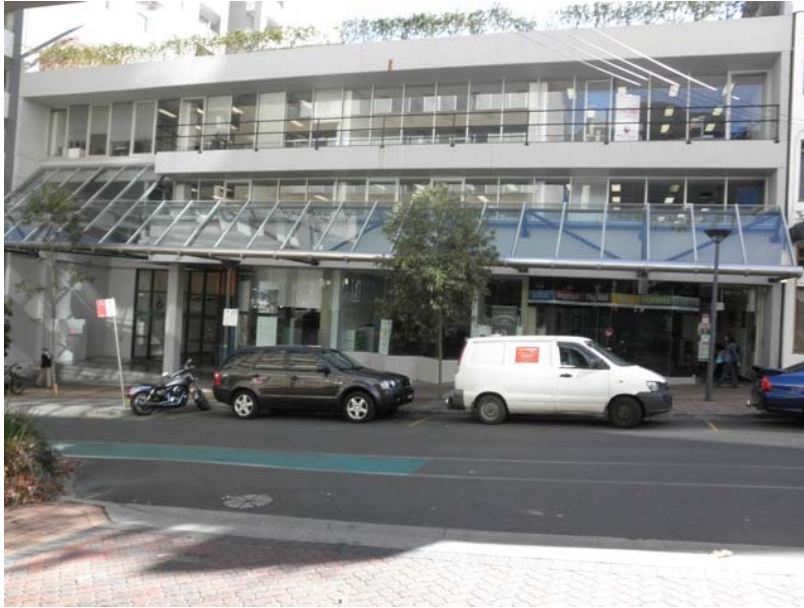
Image 4: 6-12 Atchinson St (view from Atchinson St)
