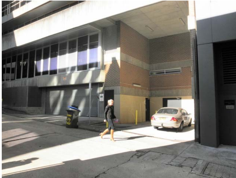
Image 6: 6-12 Atchinson St (Atchinson Lane Loading Dock)
