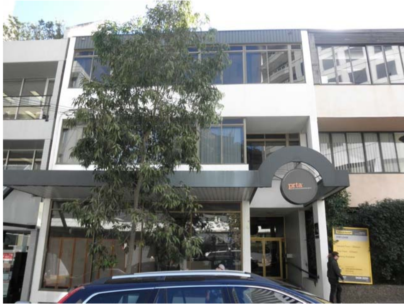
Image 8: 14 Atchinson St (view from Atchinson St)
