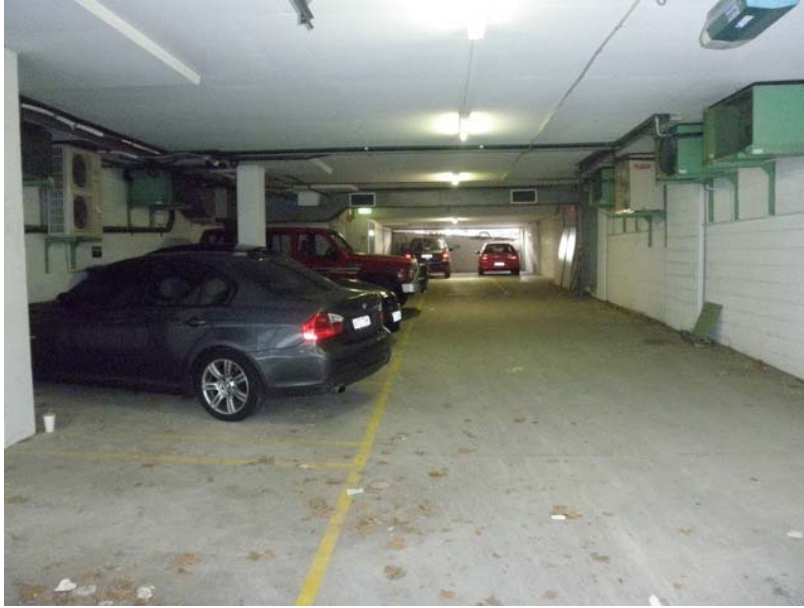
Image 10: 14 Atchinson St (Atchinson Lane car park)
