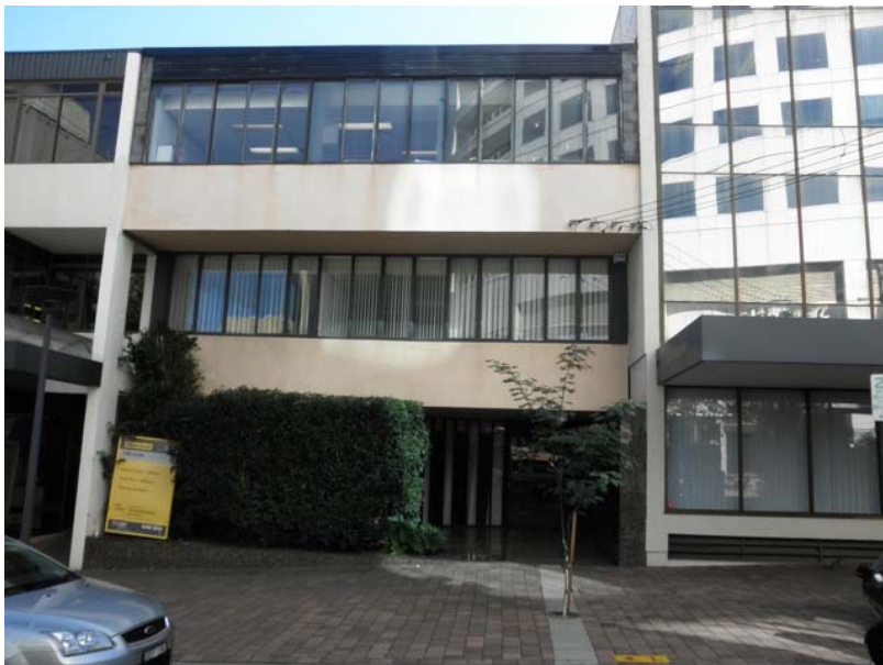
Image 11: 16 Atchinson St (view from Atchinson St)
