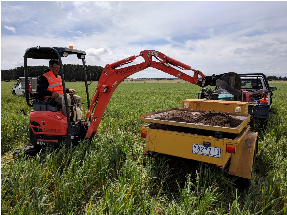
Figure 1. Excavator and mechanical vibratory screen.
