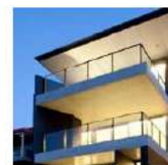
Glass Balustrade & Slab upturn
