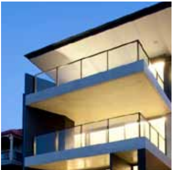
Glass Balustrade & Slab upturn
