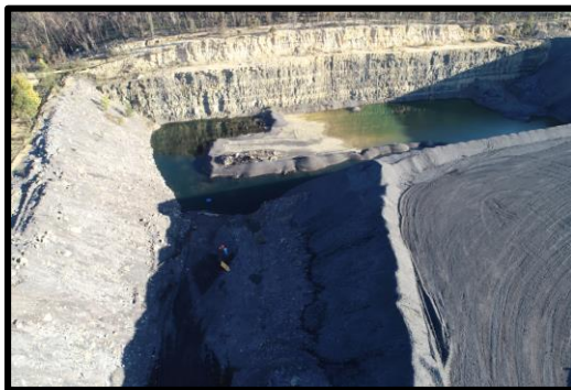
Leachate Dam – September 2020
