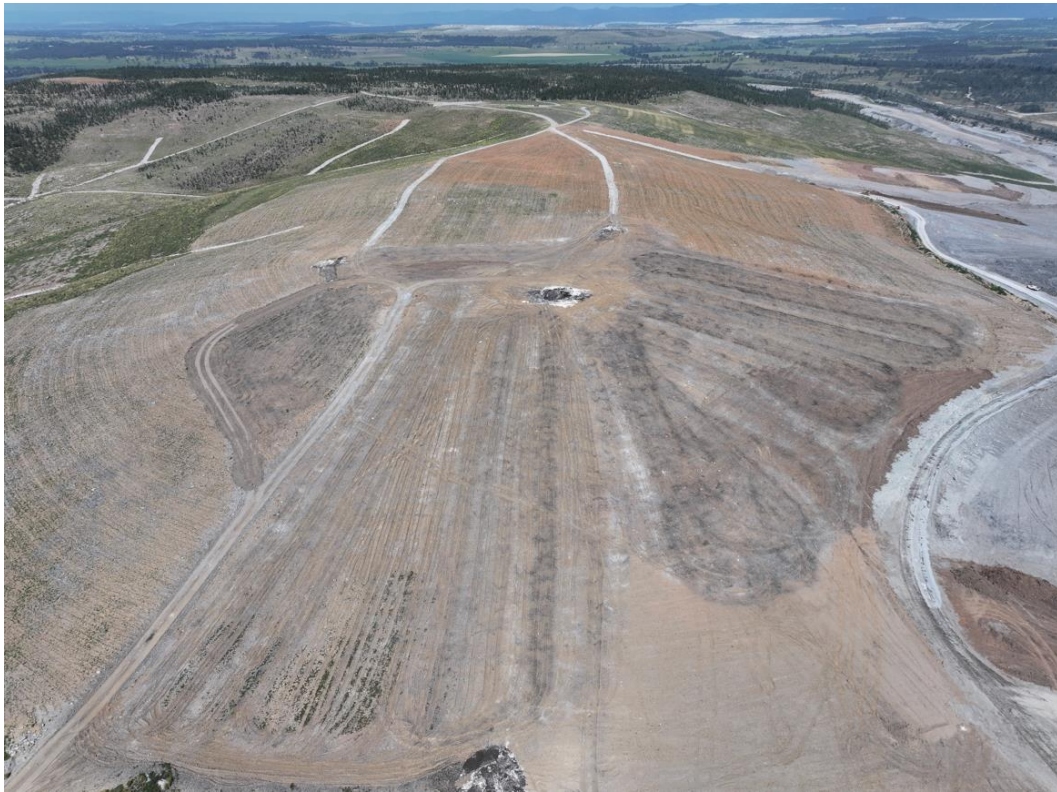
Photo 4 – Rehabilitation Progress 2024. 7 South Rehabilitation Area bulk shaping
