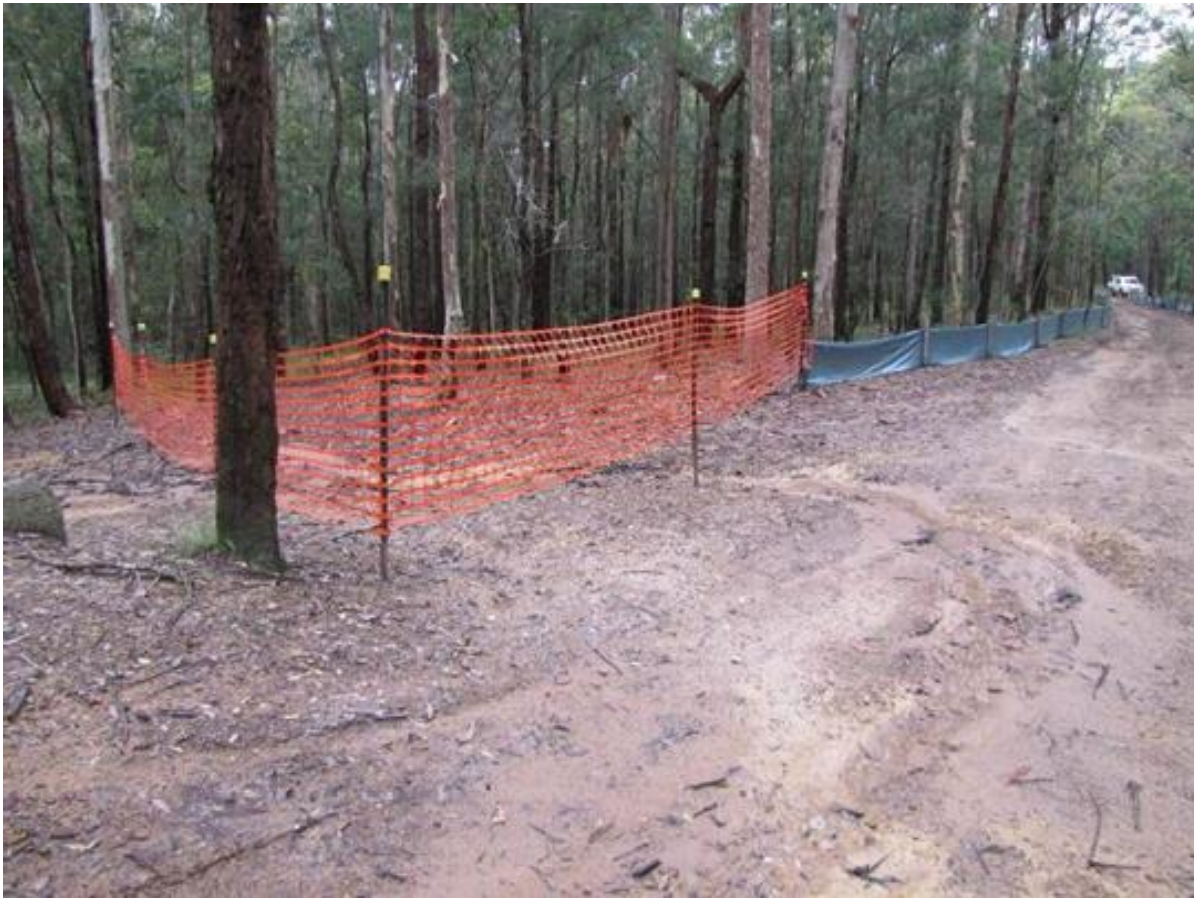
Plate 1 Example of high visibility fencing to be established around Aboriginal Sites (if required)
