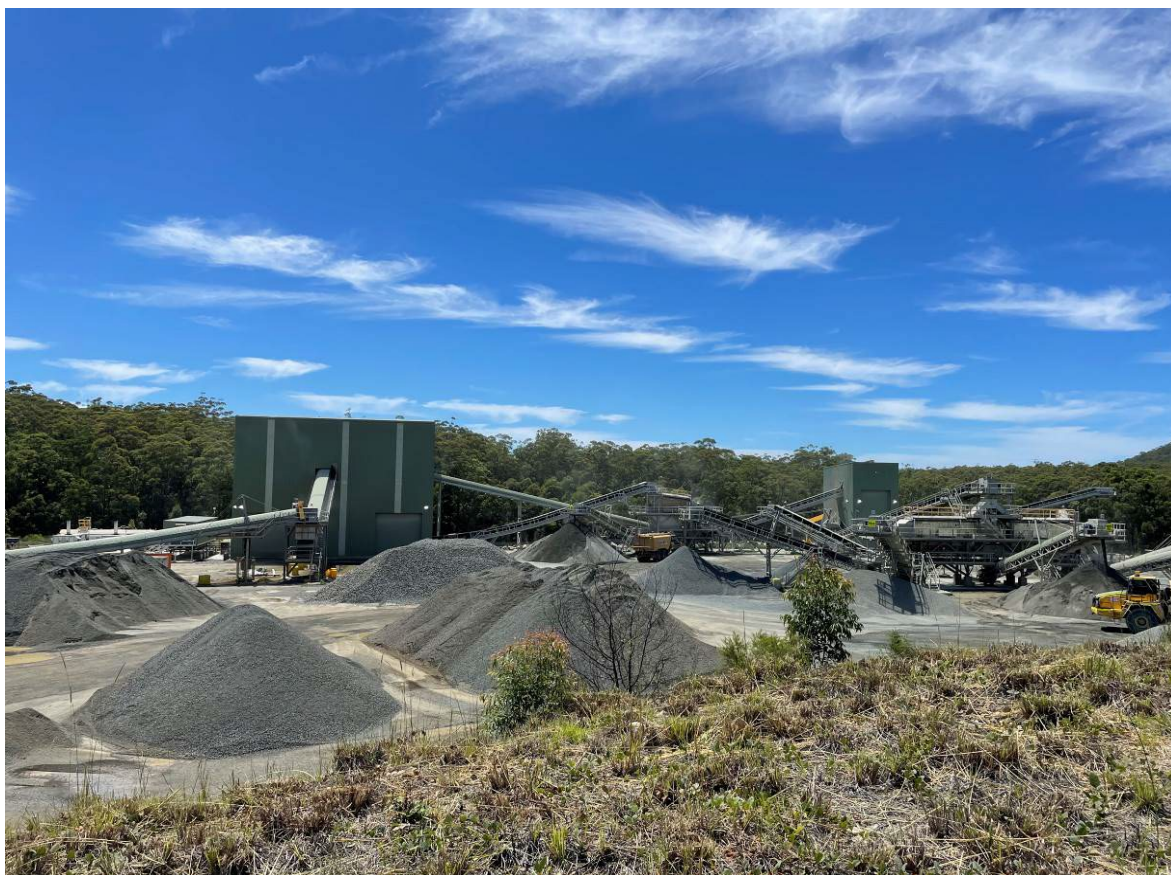
Photo 1 – Crushing Plant (January 2021)
