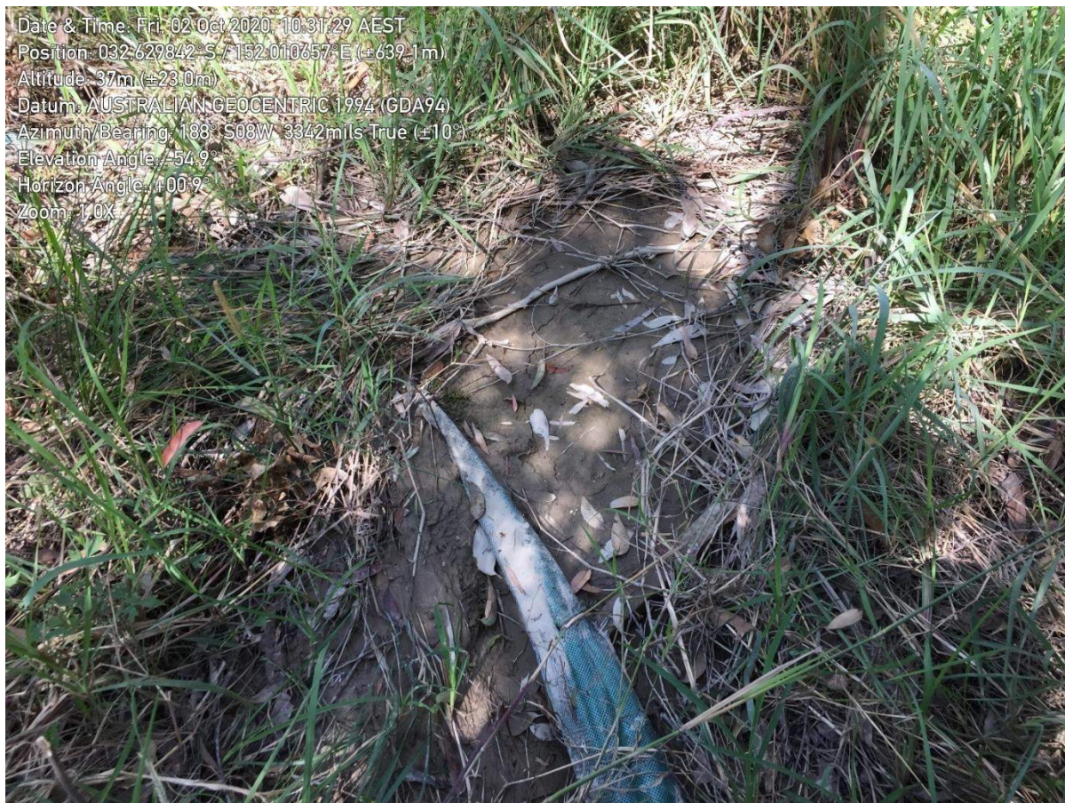
Photo 3 Sediment fencing down and overtopping within Lot 12
