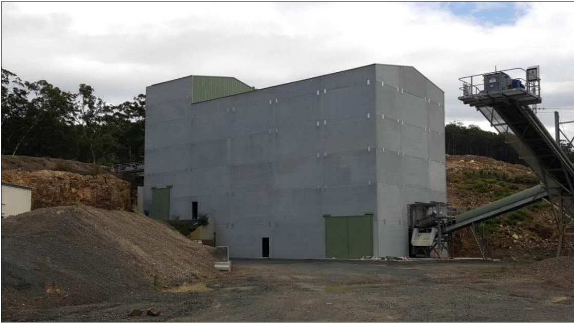
Figure 3 | Primary Jaw Crusher Enclosure
