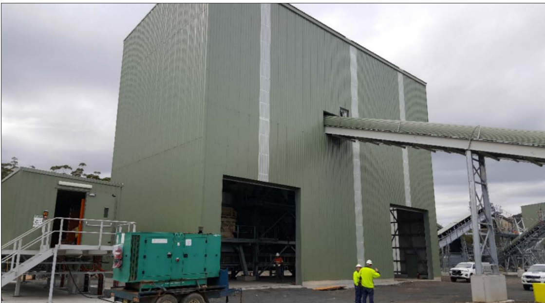
Figure 4 | Secondary Cone Crusher Enclosure
