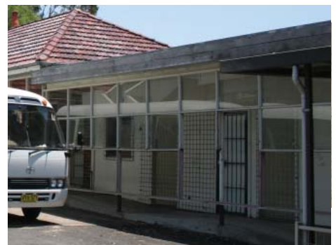
Figure 3-19: 1970s fibro extension with flat roof
